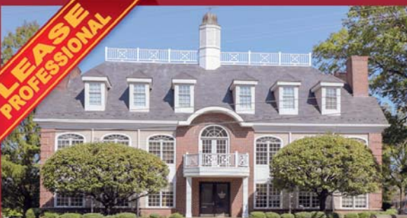
693 South State Street Newtown Twp 5,000 S.F. + Parking $10,000
